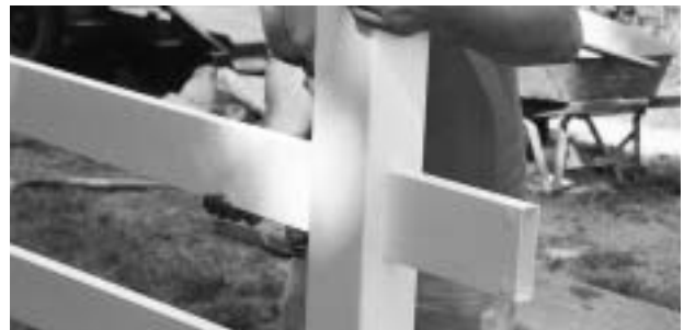
Rails are threaded through the pre-routed posts.
