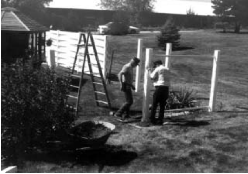
Posts are set for the entire installation.
