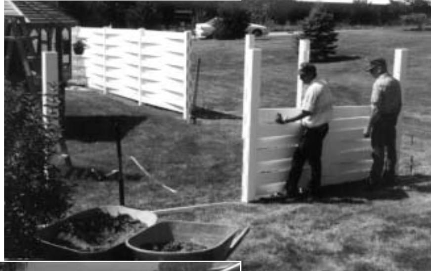
Prebuilt fence sections or horizontals are then mounted to or through the routed posts.
